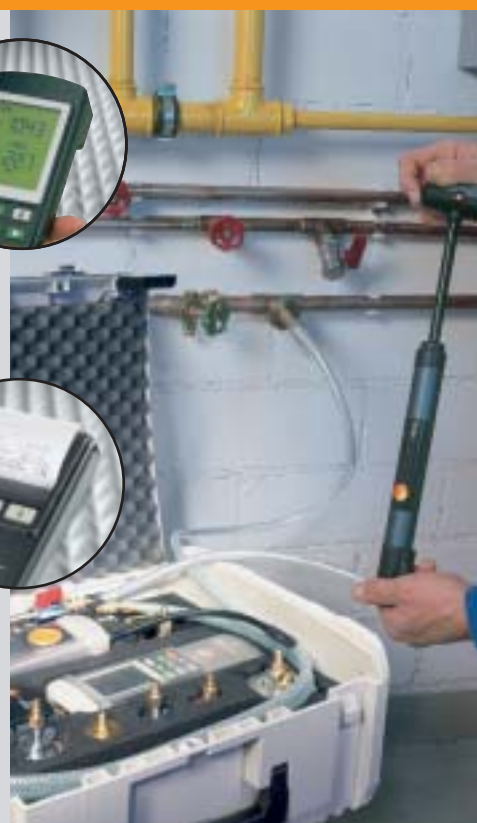
Pressure test on water pipes (3-5 bar test pressure)
