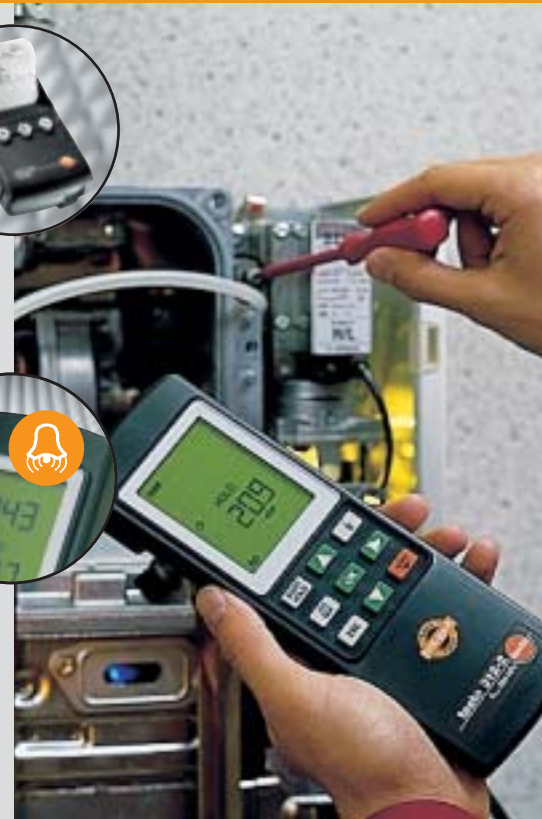
Differential pressure measurement on heating units
