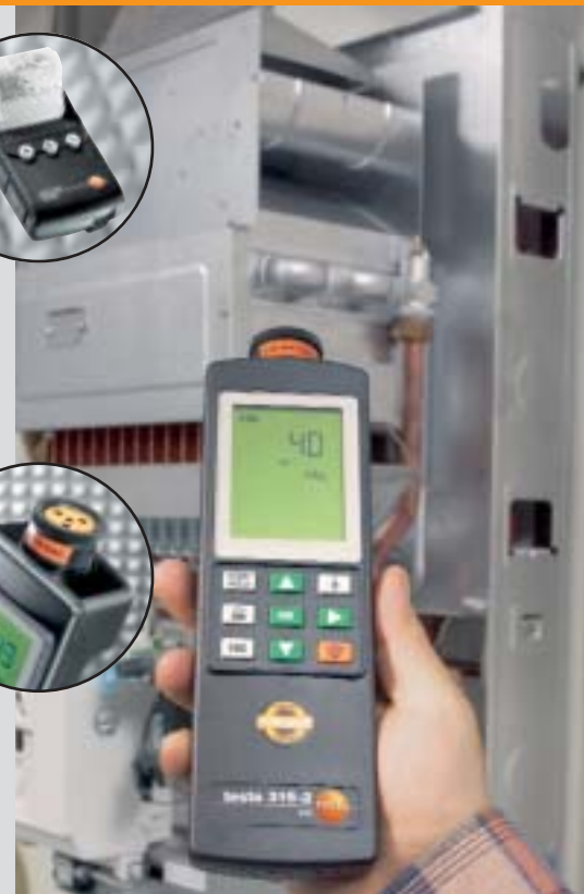
Safe CO level check
