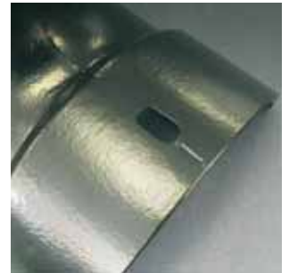
Slotted fixing holes allow for thermal movement.
