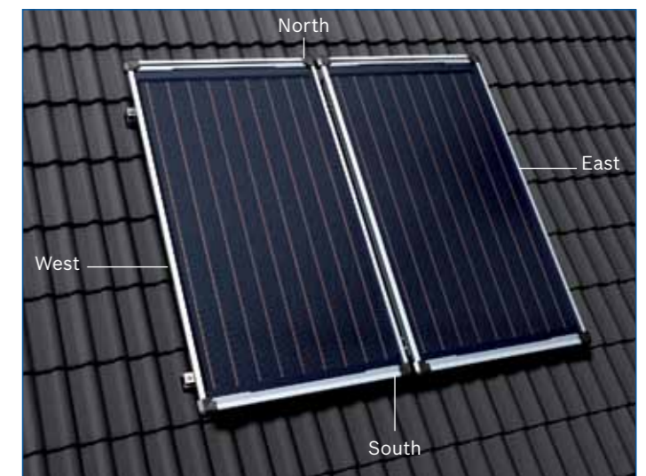
Position panels in a southerly direction for maximum potential.
