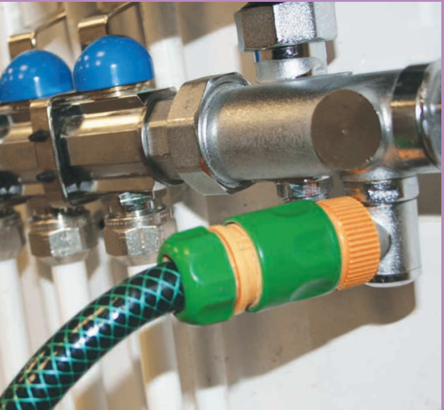
Filling, Venting and Pressure Testing
