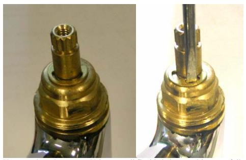
Unscrew the valve cover. Using a small flat bladed screw driver carefully prise out the existing 'E' Clip using your hand to cover the valve and clip to prevent it from flying off.
