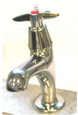
Prise off the coloured Indice with a sharp blade of a knife
