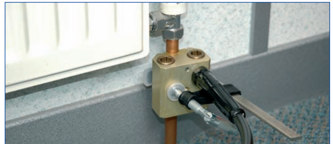
Fig. 2. Shows the compact size of the freezehead. Note the block pipe going into the back of the freezehead. This block hose should always go into the top half of the freezehead for best performance.
