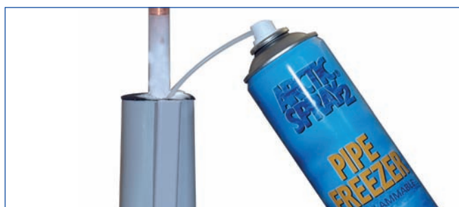
Fig. 4. Shows how to inject Arctic Spray2 into a vertical freeze point.
