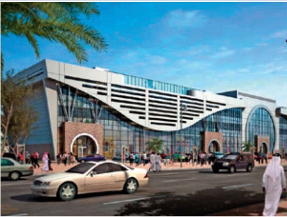
Location: Doha, Qatar Project: Barwa Commercial Avenue Application: AB-QM for cooling
