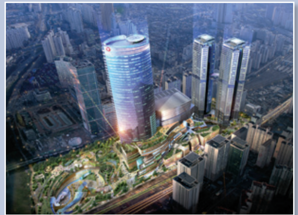
Location: Seoul, South Korea Project: D-Cube city and shopping mall Application: AB-QM for heating and cooling
