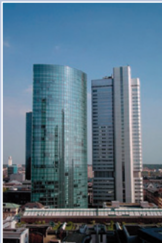
Location: Frankfurt, Germany Project: Silver Tower Application: AB-QM for heating and cooling
