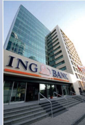
Location: Istanbul, Turkey Project: ING bank Application: AB-QM for heating and cooling
